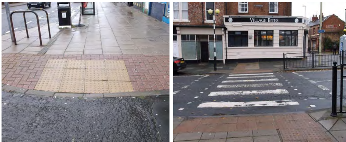
Figure 3.1 – Examples of Pedestrian Facilities in the Area: Colour Contrast and Tactile Surfaces on Dean Road (left) and Zebra Crossings and Guardrails on Imeary Street (right)
